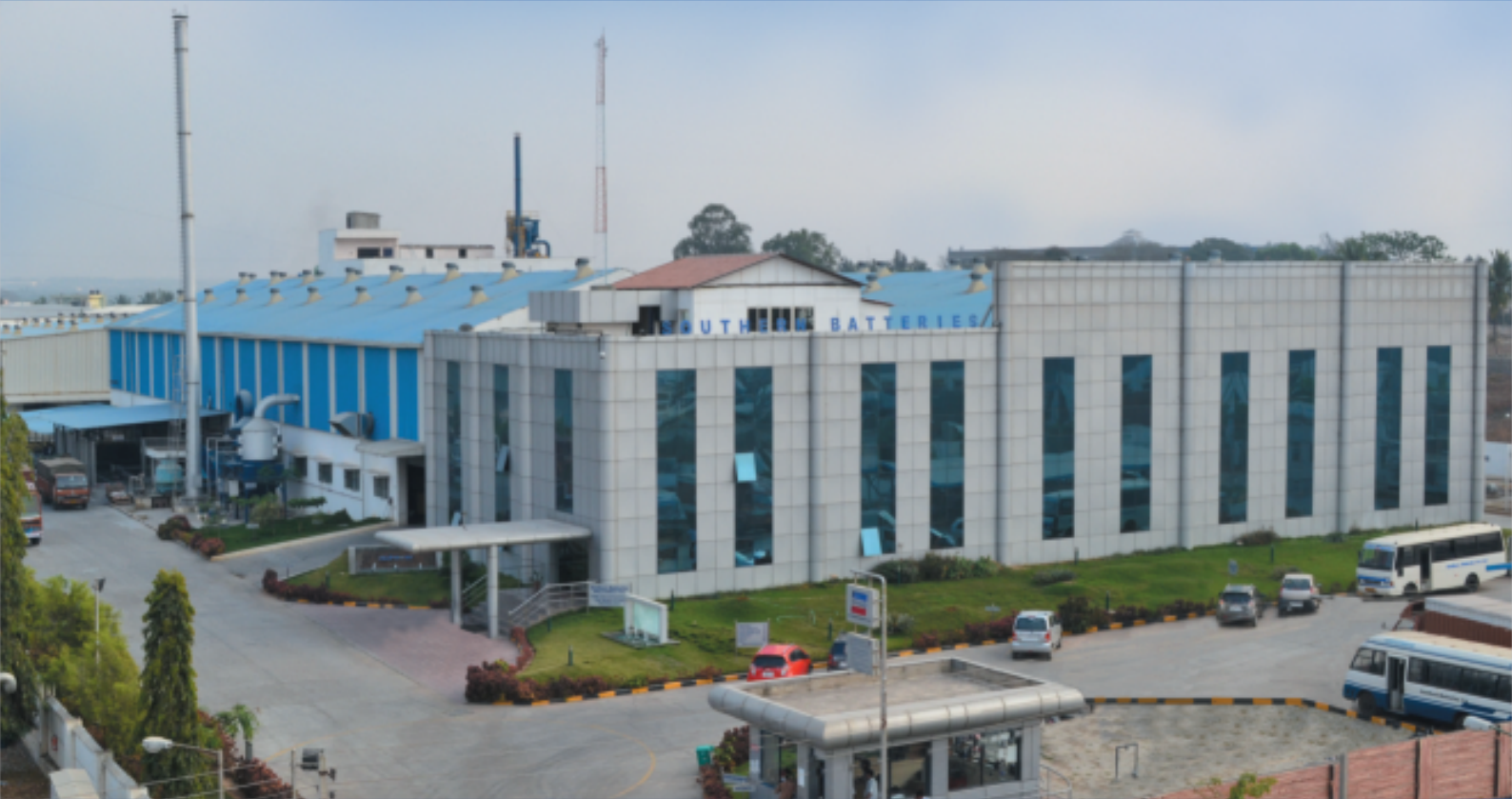
View of our corporate office and two manufacturing units at Jigani, Bangalore
